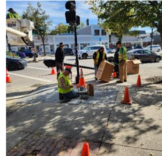
Crew getting ready to set décor light.
