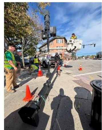
Street light replacement
