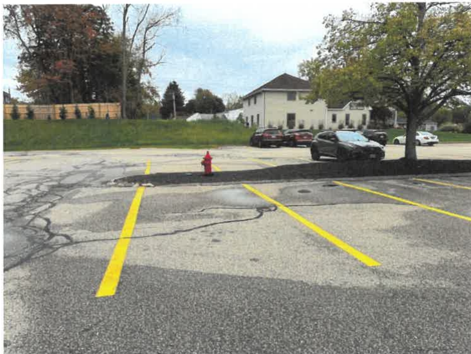
Photo 8: Existing parking island with hydrant to be cut back
