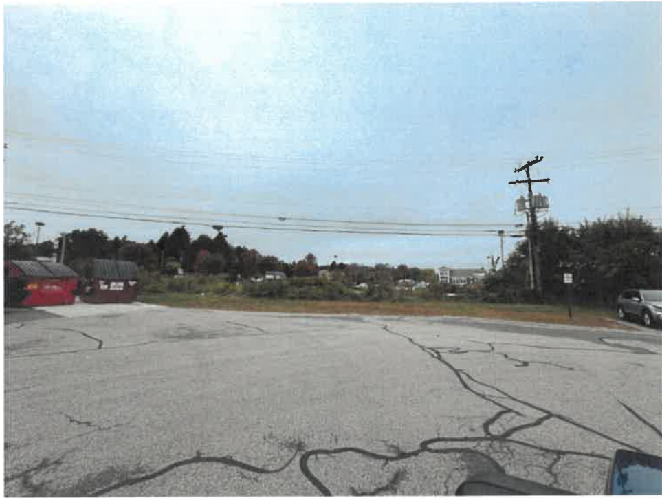
Photo 11: Location of proposed driveway access to Shaw's from Hannaford access road, facing northwest
