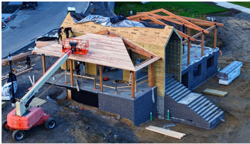
Pavilion Roof Install
