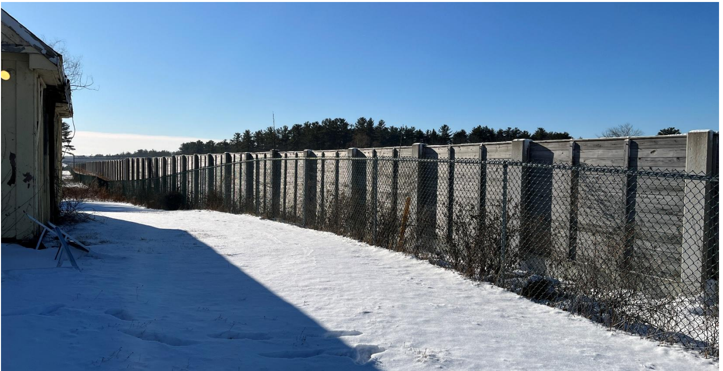
View of the right side of the property, showing the sound barrier, chain-link fence, and part of the utility easement.
