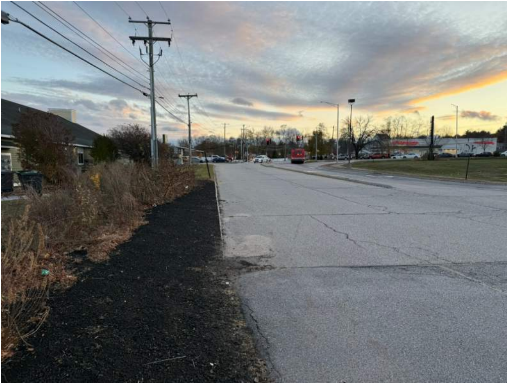
Photo 1: Looking from proposed driveway connector location toward Central Ave.
