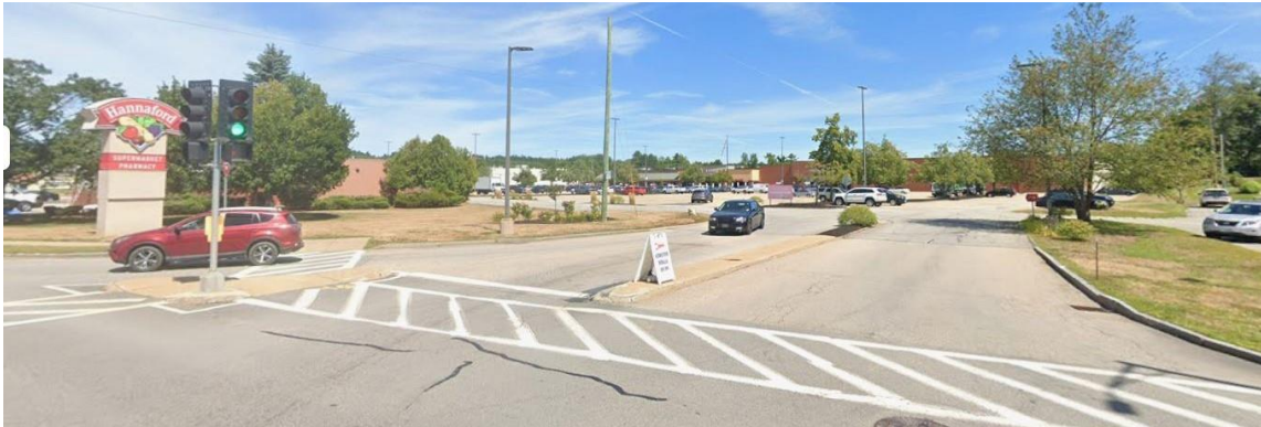
Central Avenue intersection
