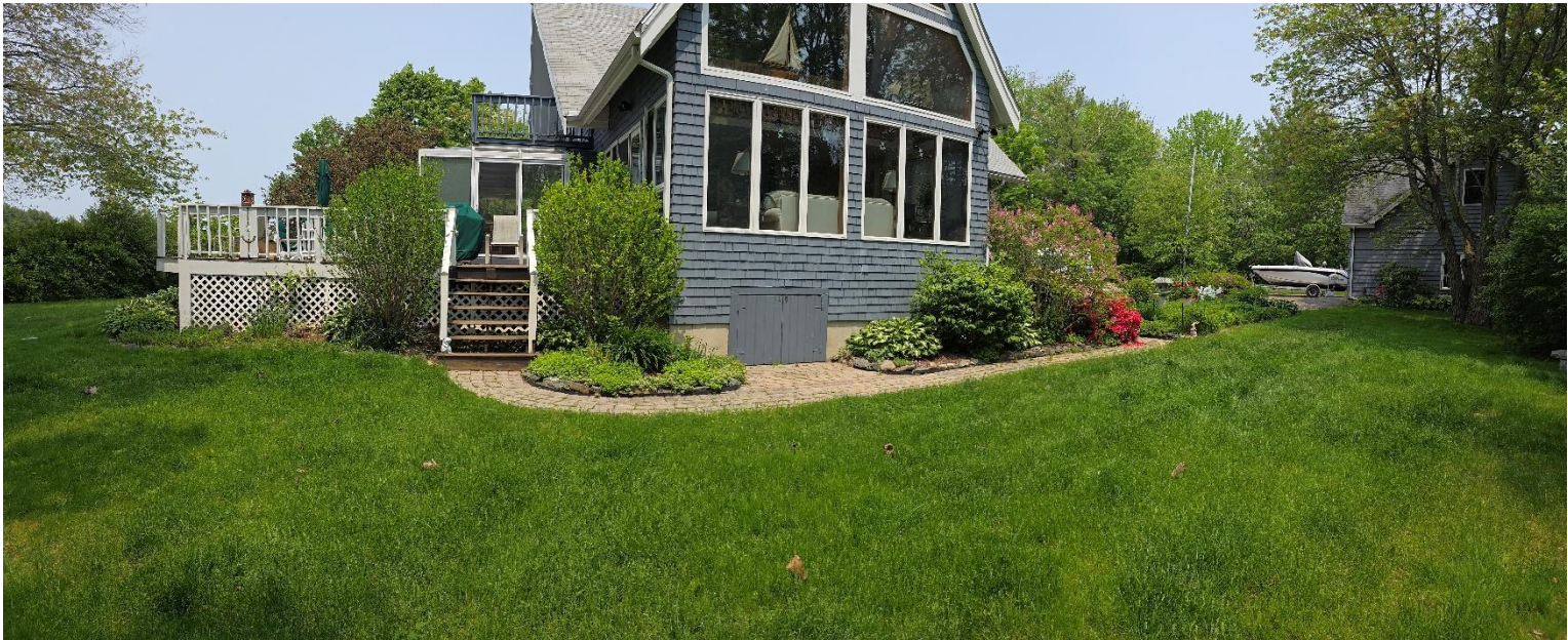
Photo 4. The sunroom and deck, viewed from the side.
