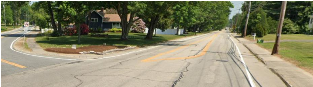
Facing north at Bellamy Rd. The yellow striping across the unmarked crosswalk is confusing and discourages pedestrian access.
