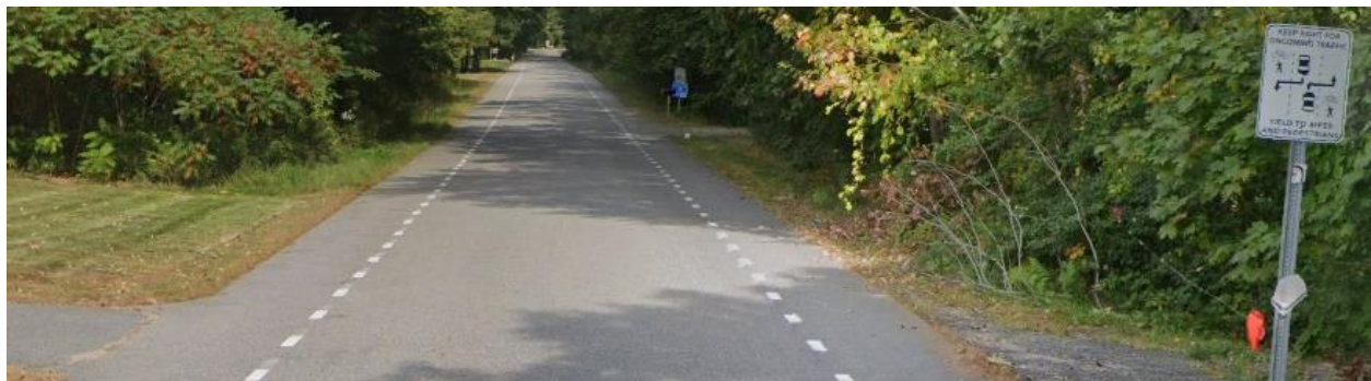
Eastern Rd near ME-207, Scarborough ME (Sep-2024). 5' edge lanes, 14' 06" center lane. 23
