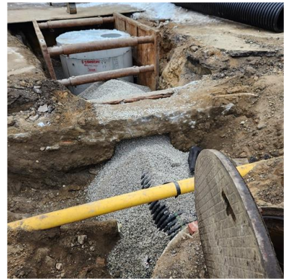
Hale & Locust Drainage Project
