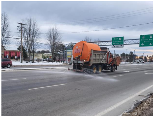
Crews pretreat the roads with Brine to reduce the amount of salt applied to the roadways.
