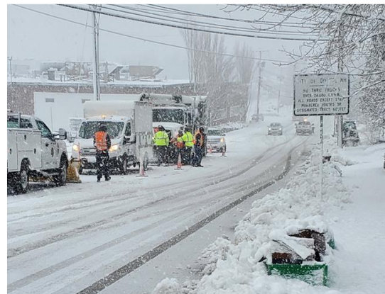
Utility crews working to address a sewer back up in the middle of a storm while sidewalks are being plowed by CS staff.
