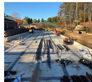
Jenny Thompson Renovation Progress
