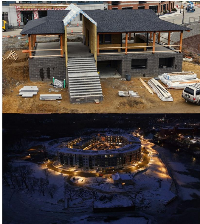
The Waterfront comes alive at night with new street lighting as the Nebi Park pavilion keeps moving along.
