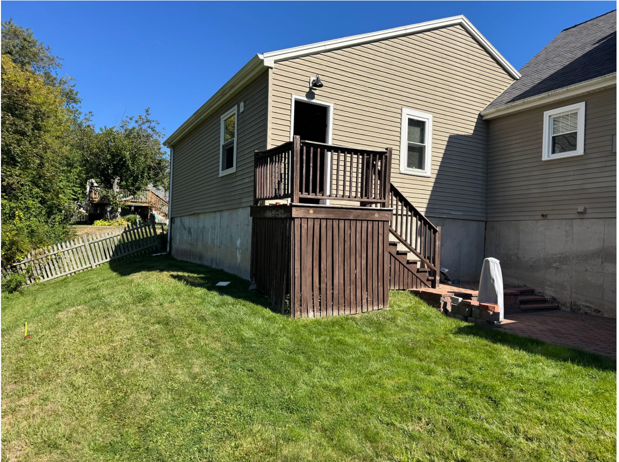
Photo 2 – Existing Conditions Photos
