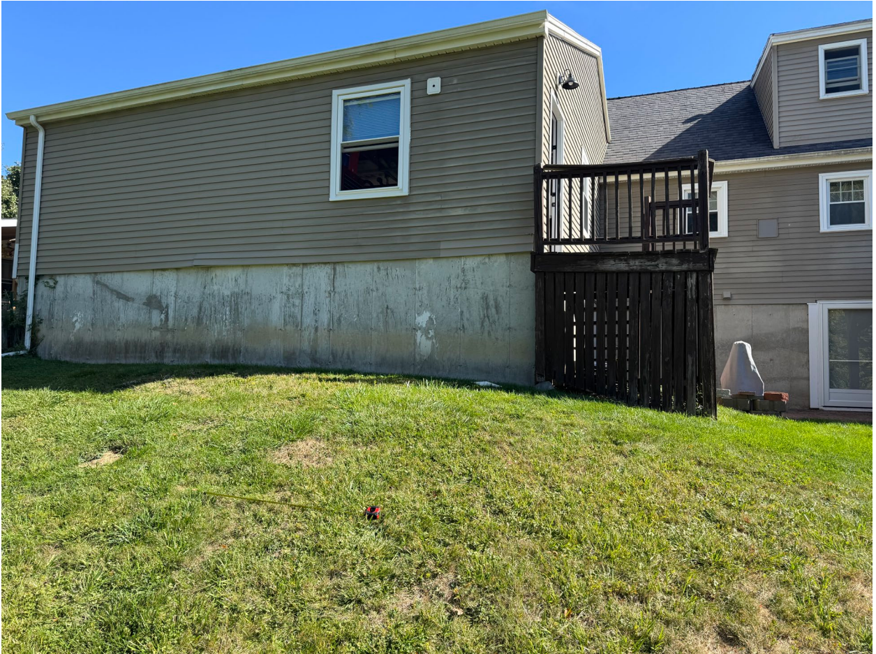
Photo 3 – Existing Conditions Photos
