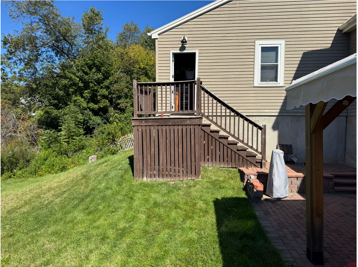
Photo 5 – Existing Conditions Photos
