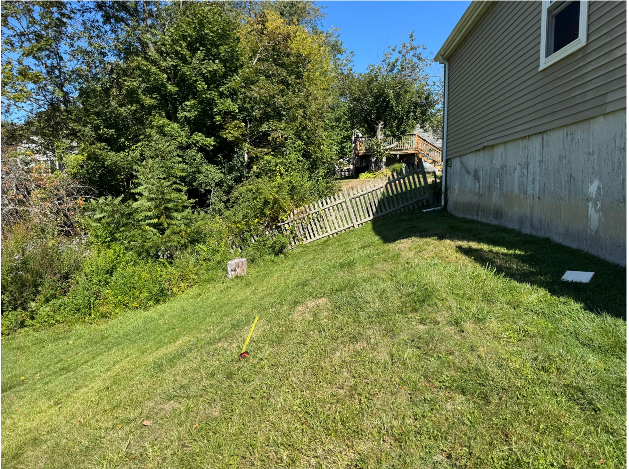
Photo 4 – Existing Conditions Photos
