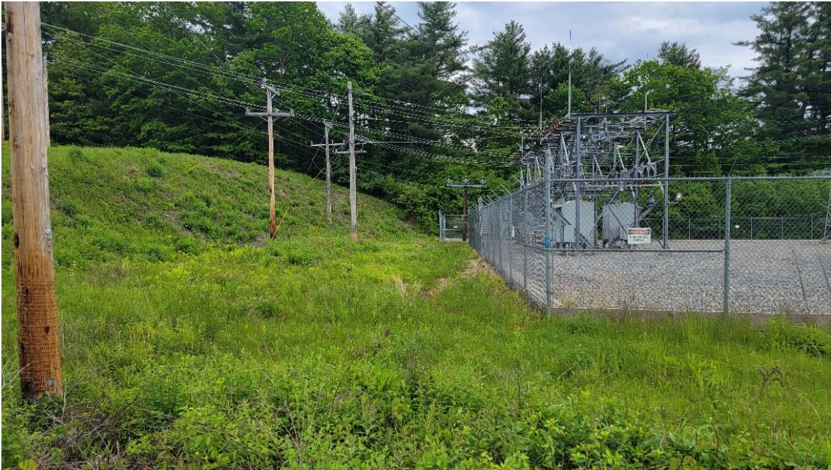
Photograph No. 1: Looking east at the location of the proposed wetland impacts at the north side of the substation.
