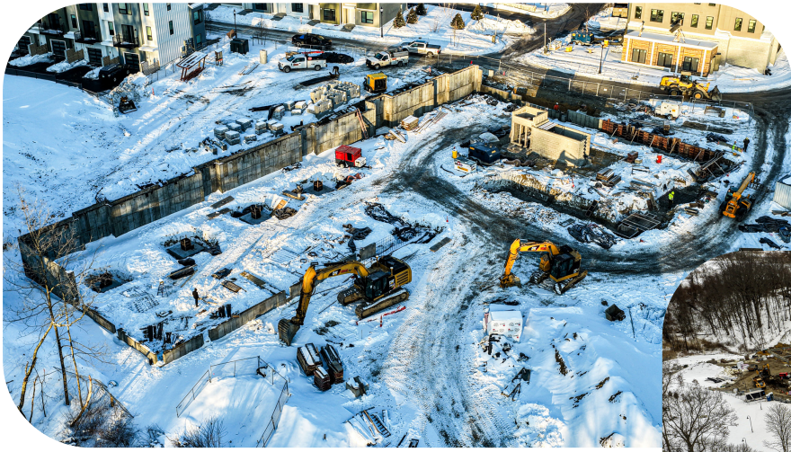
Building F Foundation
