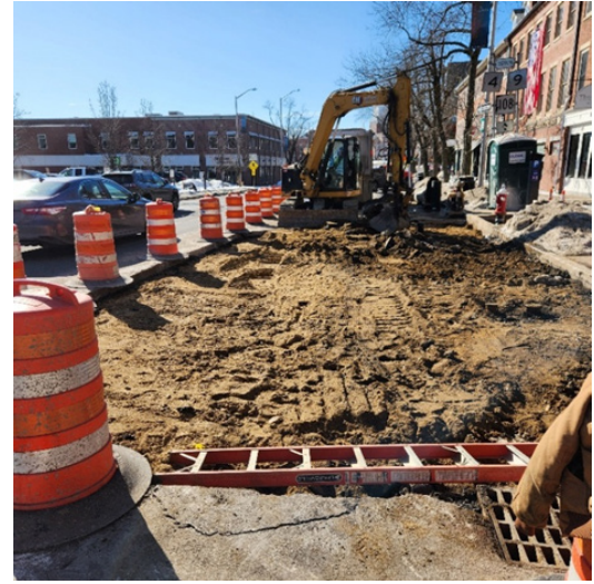
Right: Pavement removal on Central Ave to accommodate a new pedestrian bump-out.
