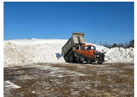
Dumping snow at the Maglaras Park temporary snow dump before heading back for another load.
