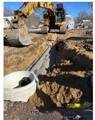
Drainage structure installation in Court St. page 12 of 71
