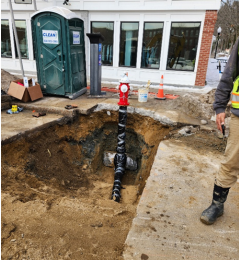
Left: A new hydrant has been installed near a new pedestrian curb bump-out.
