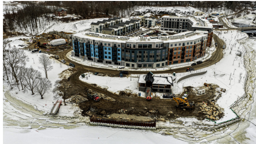
Progress on the Pavilion building and granite toe wall.
