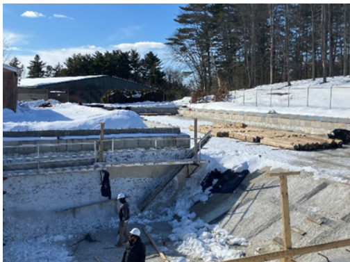
Jenny Thompson Pool renovation as of 02.26.2026
