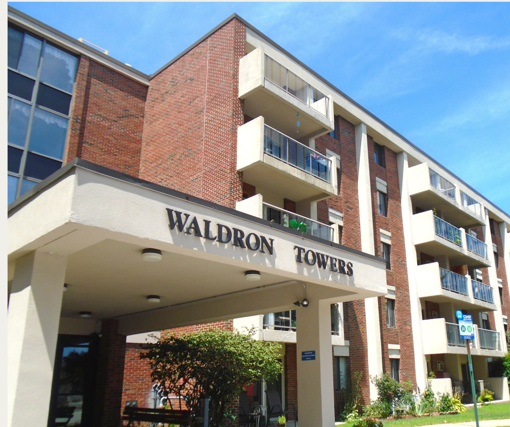
Pictured: Waldron Towers
