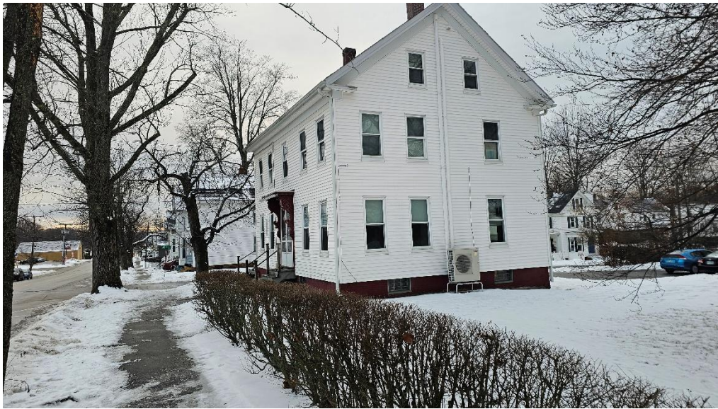
Photo #1- Existing structure at the south corner of the subject parcel. (January 07, 2026)
