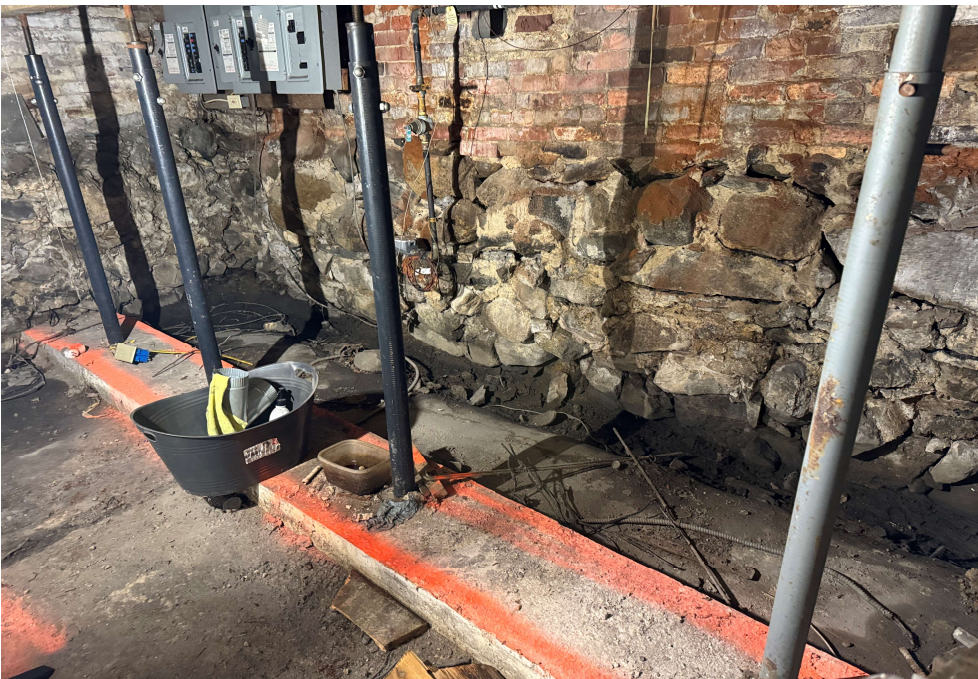
Basement, note stone foundation wall with scour ditch at base
