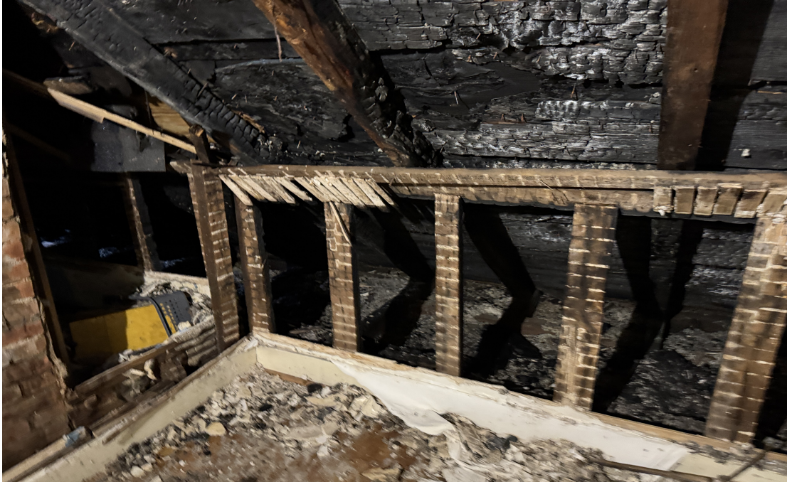
Roof planks and rafters
