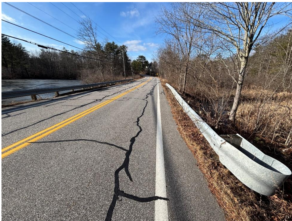
Photo 5 – Guardrail and Wetland Area on North Side of County Farm Road
