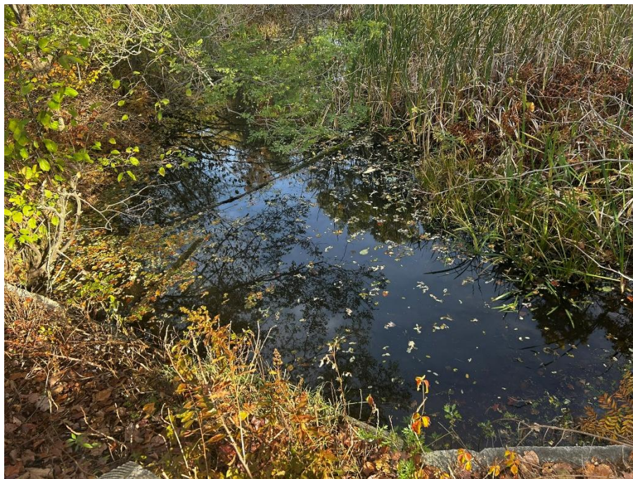
Photo 4 – Wetland Area at Inlet of Granite Box Culvert in Unnamed Stream
