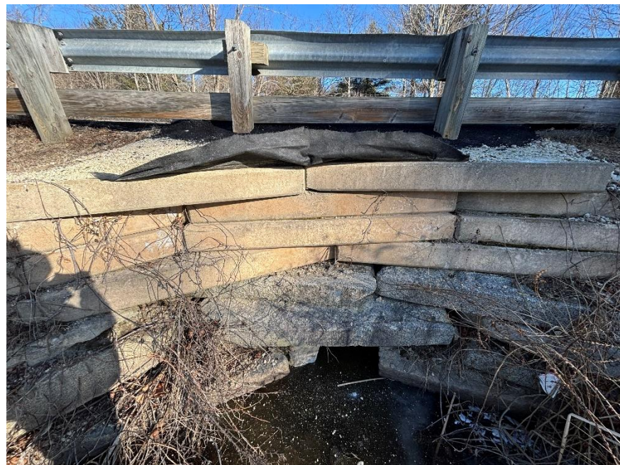
Photo 2 – Outlet of Granite Box Culvert w/ Granite & Concrete Headwall in Unnamed Stream at County Farm Road
