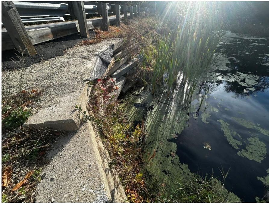
Photo 3 – Outlet of Granite Box Culvert w/ Granite & Concrete Headwall in Unnamed Stream at County Farm Road
