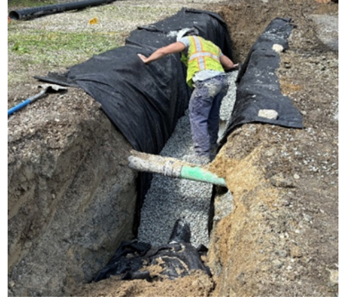
New underdrain pipe with fiber mesh wrap and crushed stone for support.
