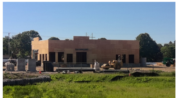
McDonalds on Grapevine Drive construction progress
