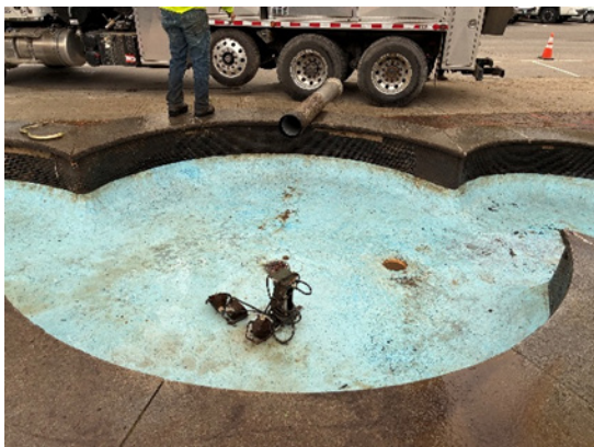
Crews using the vector truck to remove soil.
