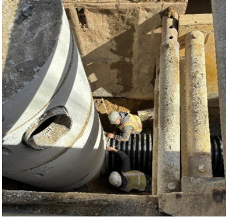
Large diameter drain manhole install.
