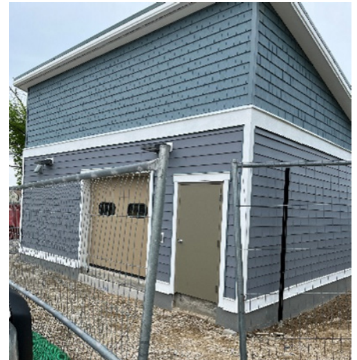
Pool maintenance building.
