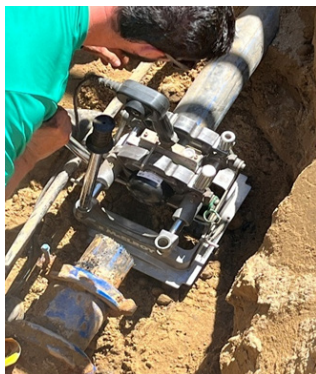
Utilities crew completing the install.
