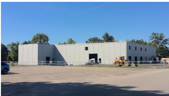
34 Industrial Park site work progress
