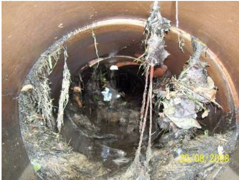
Figure 2-1 Condition of Aging Stormwater Infrastructure
