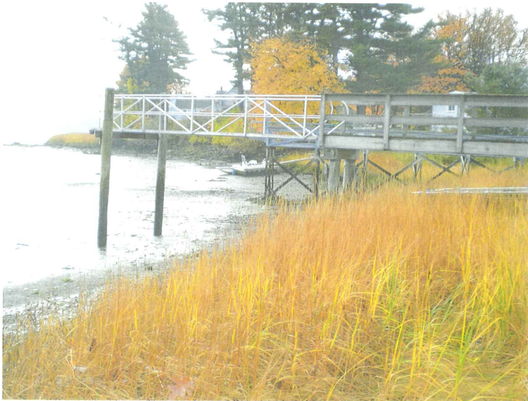
PHOTO #4: LOOKING SOUTH AT ADJACENT DOCK UNIT A
