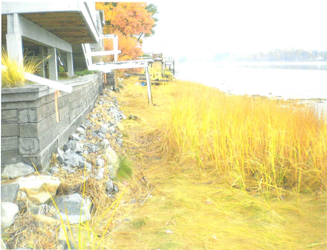
PHOTO #2: LOOKING NORTHEAST AT EXISTING REMAINING DOCK
