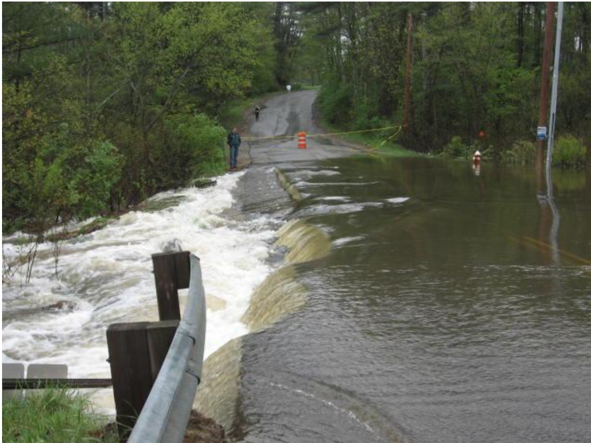
Flooding in the City of Dover; 2007
