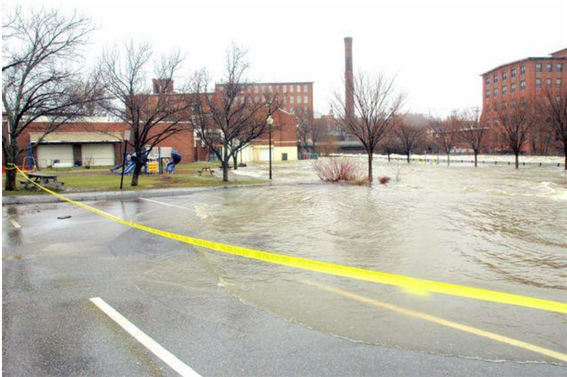
Cochemo River flooding in downtown Dover; 2007
