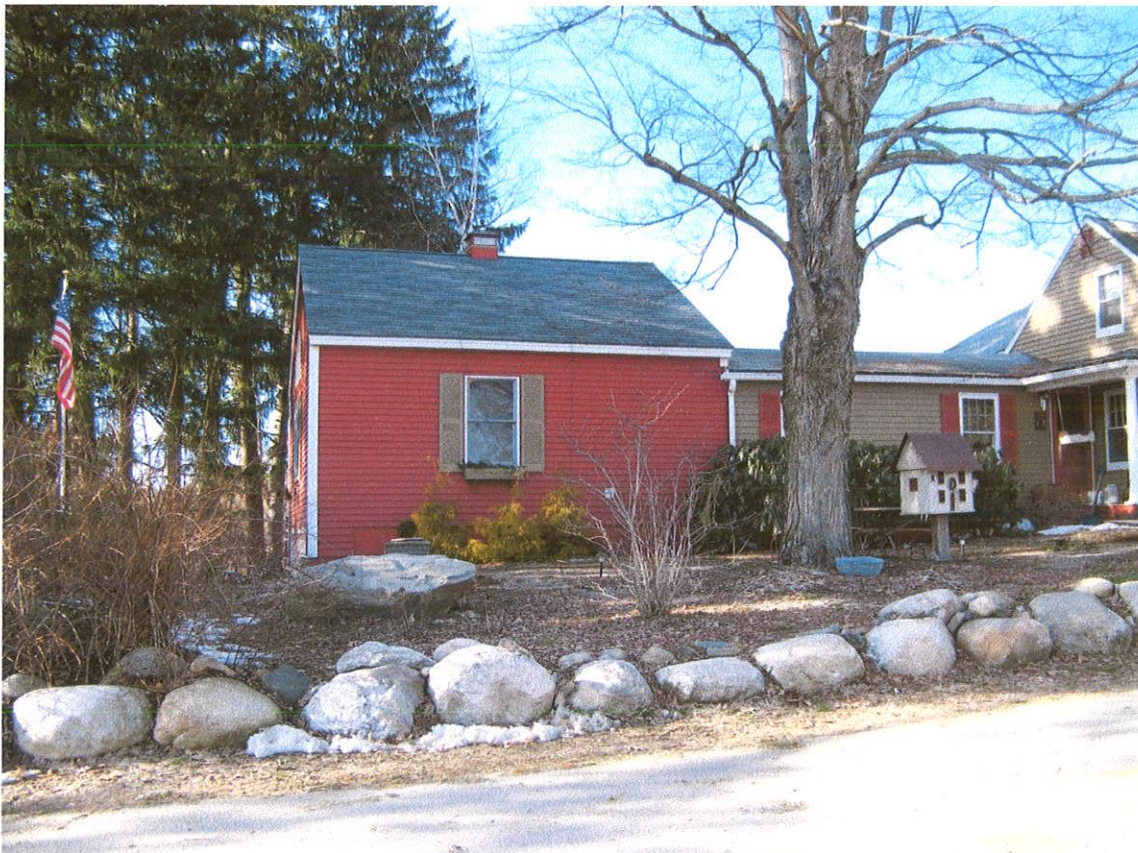
Photograph #4 – Existing Garage & House
