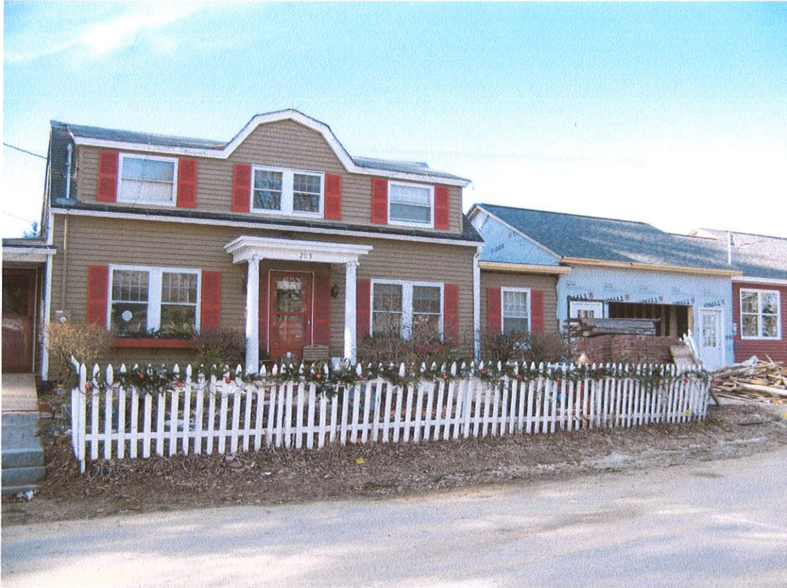
Photograph #1 – Existing House & Addition
