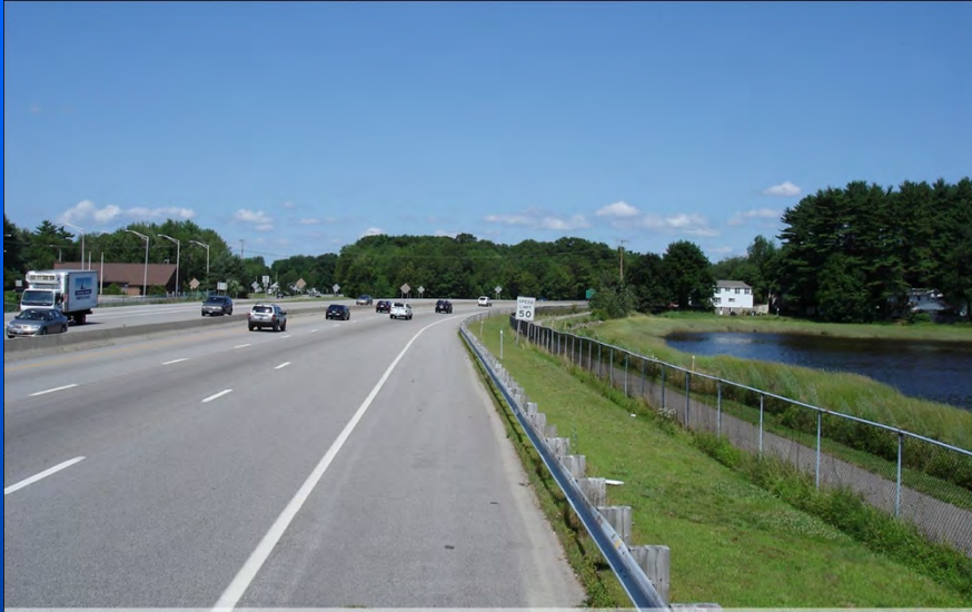
Pomeroy Cove - Looking Northwest from Exit 5 On-Ramp
