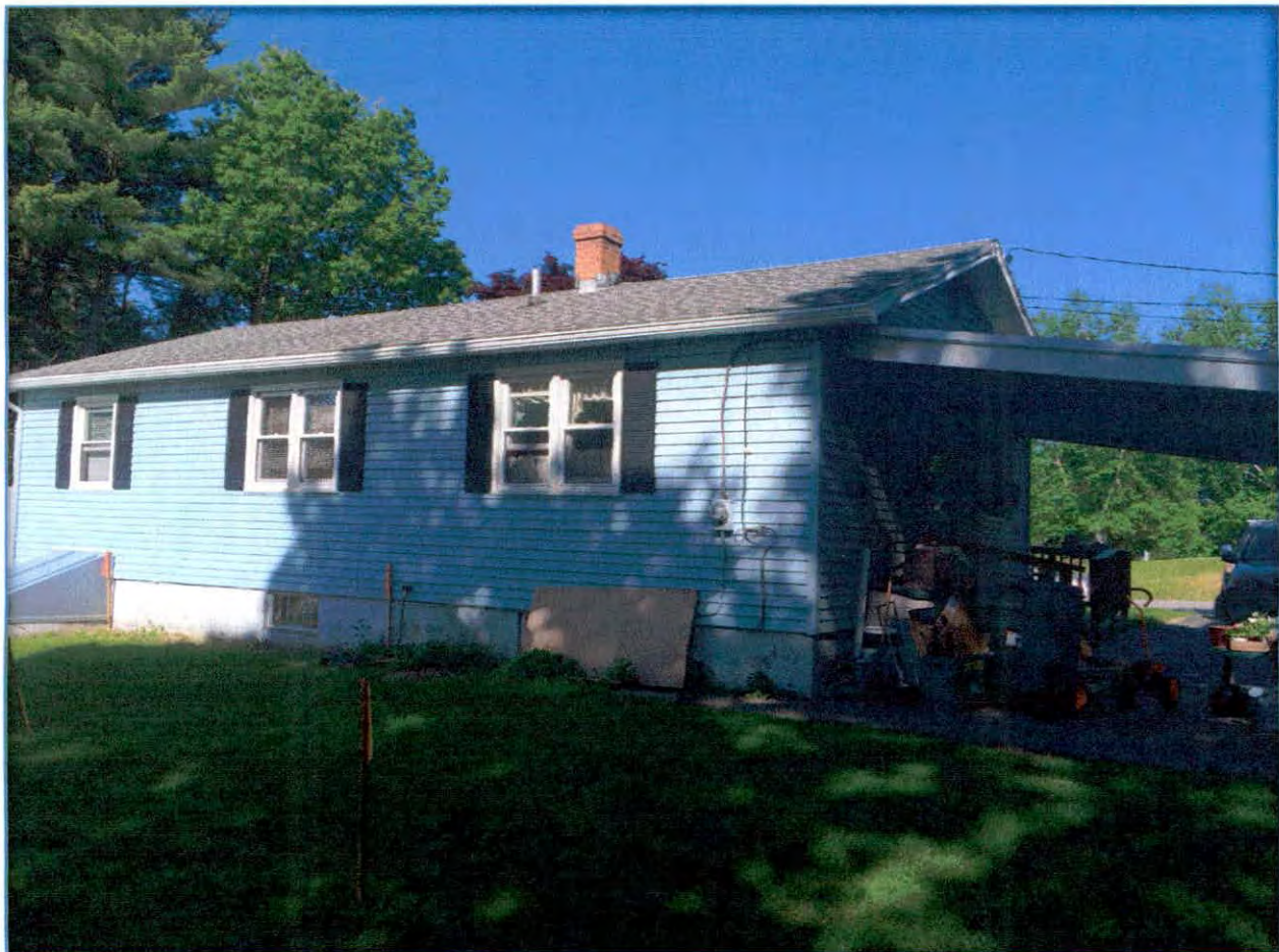
Back of House with views of carport, rooflines, and layout for addition
