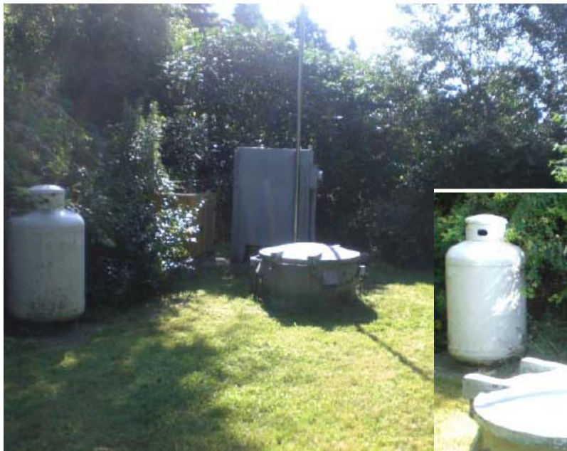
Leighton Way Pump Station to be Replaced
