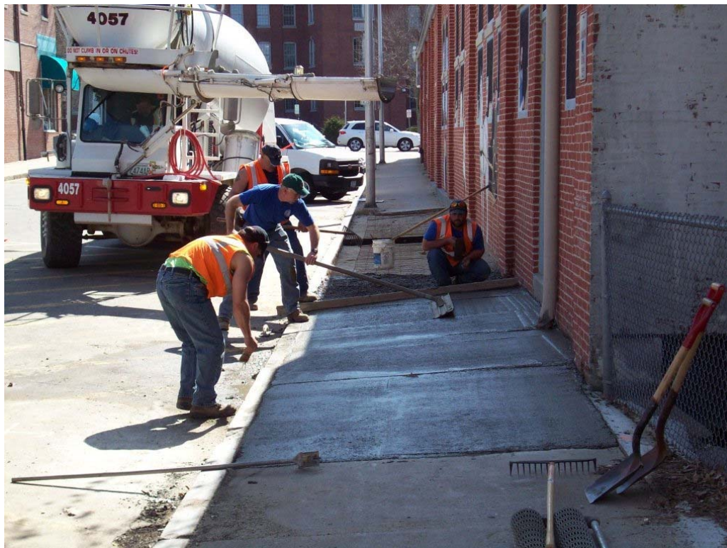
A Sidewalk Being Installed
