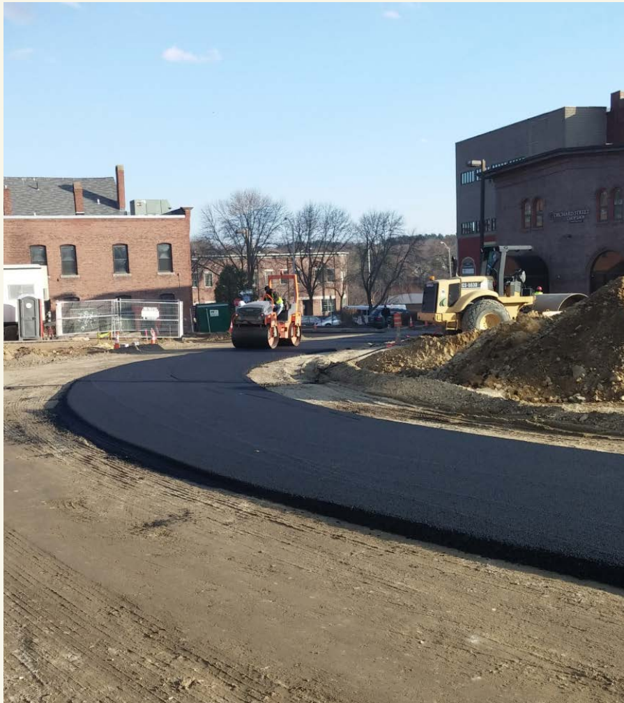
Crews paving the newly aligned Orchard Street
