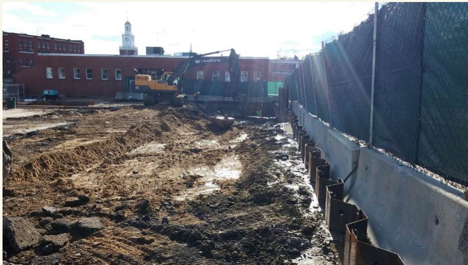
Crews excavate along Chestnut Street.
