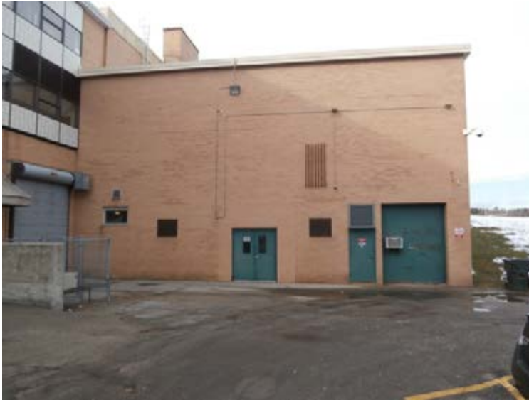
5. North side of 1966 building – low roof locker room wing.
