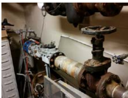
Original building water service & meter
