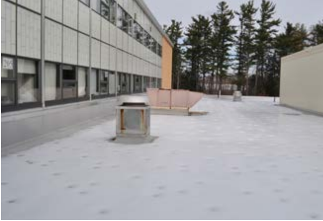
View of Roof with snow cover
