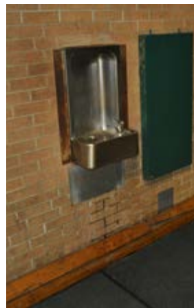
Drinking Fountain, Aged Base Board & Cracking CMU
