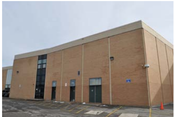
Exterior Wall System 1 - Brick Veneer
