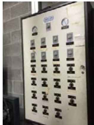
Existing CTC Building ATC System Pneumatic Compressor and Control Panel
