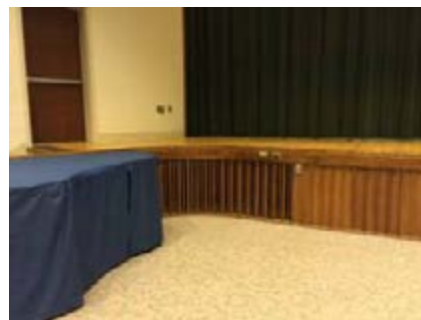
Auditorium - Return Register
