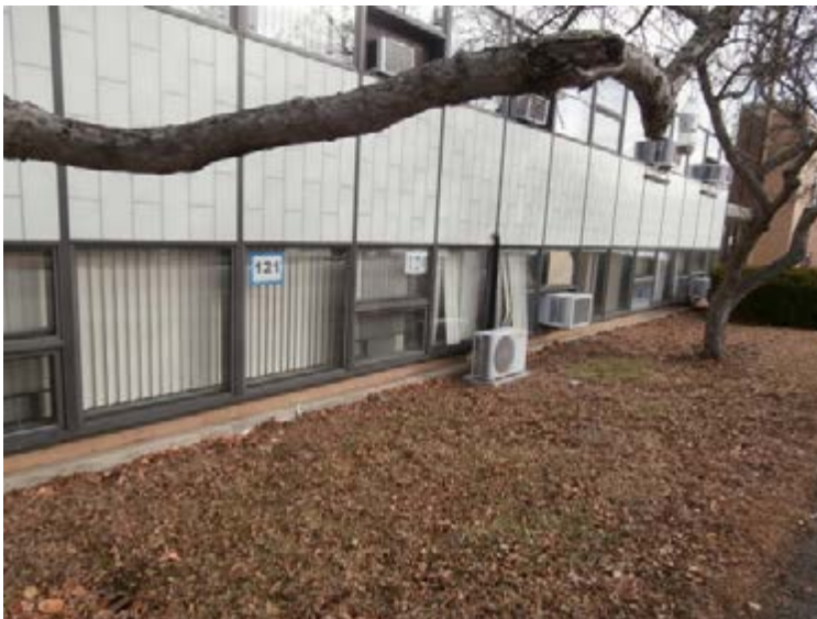
2. 1966 Classroom wing: South side window sill elevation near grade.
