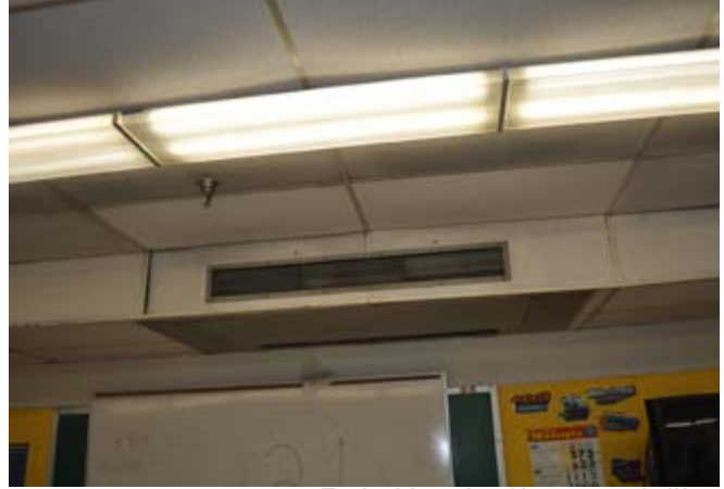
Typical Interior Classroom Ceiling
