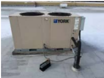
Administration Area ACC Unit
