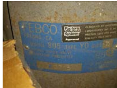
Double check valve assembly
