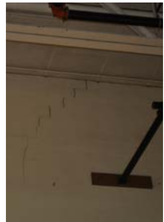
Drinking Fountain, Aged Base Board & Cracking CMU
