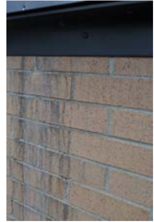
Stained Brick Under Curtain Wall System
