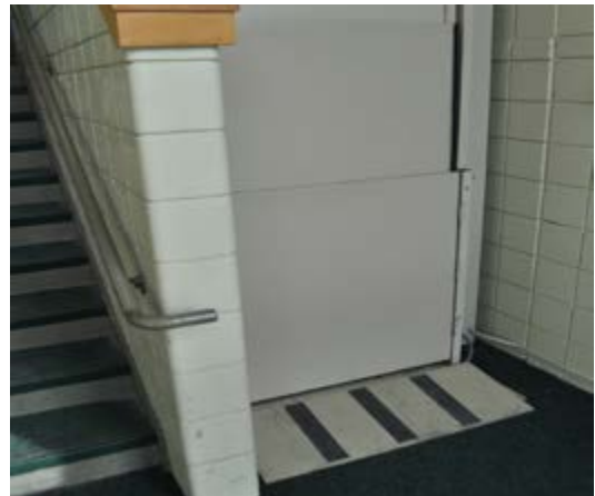
Lift at CTC Entrance
