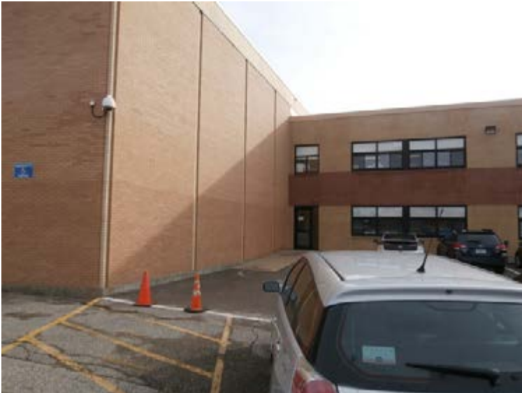
8. West elevation: 2002 addition (right) meeting auditorium wall.
