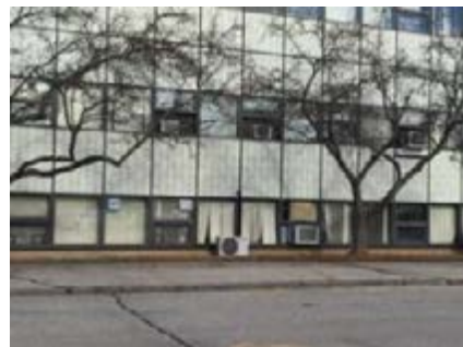
Window AC Units
