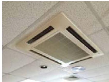
CTC Dining Room Ceiling Ductless AC Unit (typical of 2)
