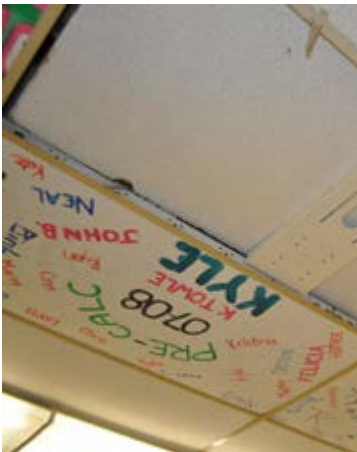
Typical, Painted Ceiling Tiles
