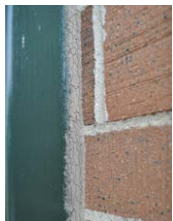
Cracked Sealant
