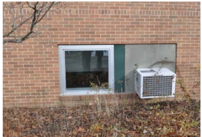
Windows Located at Grade
