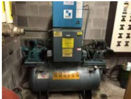
Existing CTC Building ATC System Pneumatic Compressor and Control Panel
