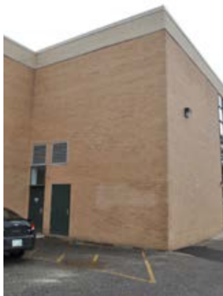
Visible Efflorescence
