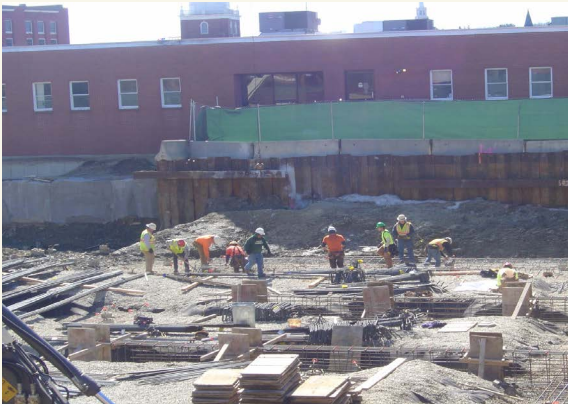
Crews install rebar for police building foundations
