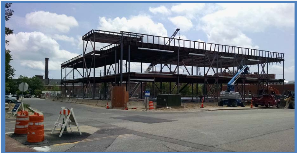
View of police facility construction site from Chestnut Street.
