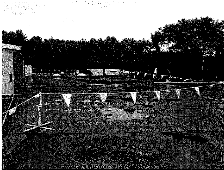
Garrison original roof to be replaced
