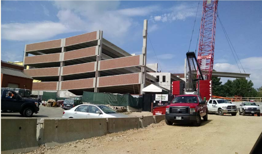
View of the southern side of the parking garage
