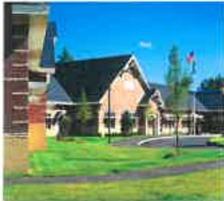
Idlehurst Elementary School
