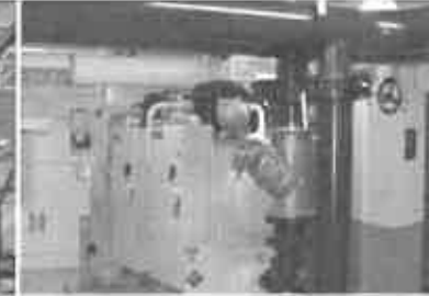
Magnetic Frictionless Chillers
