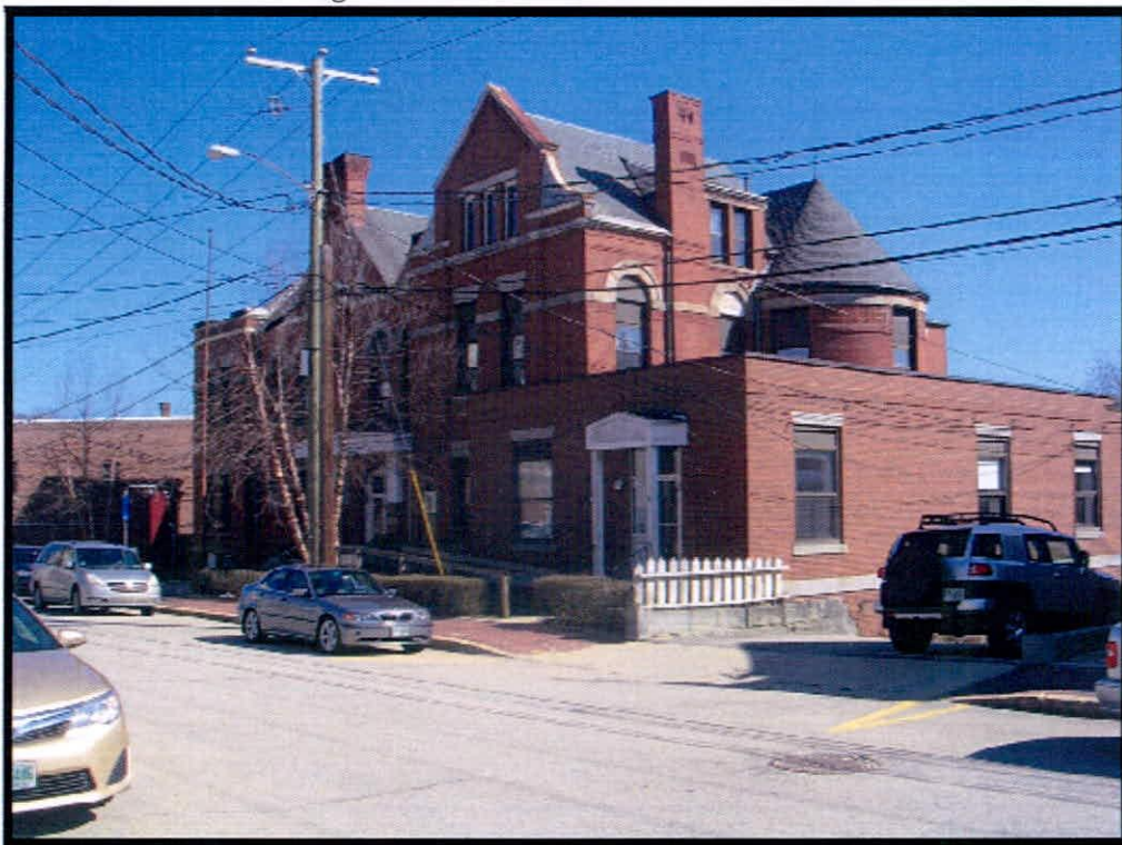
Photo 6 – Existing annex elevation. (4/5/16)
