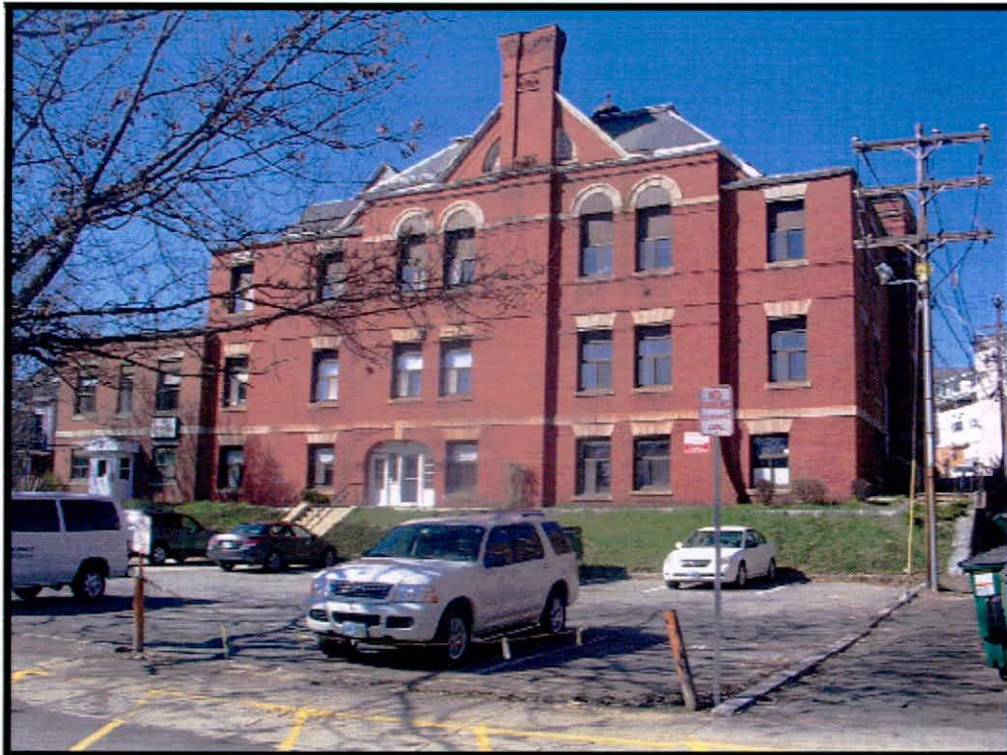
Photo 4 – Existing First Street elevation. (4/5/16)
