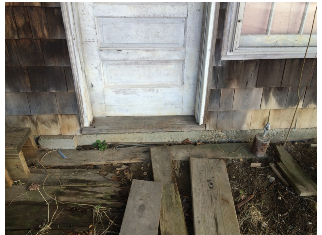
Grade at Basement Door
