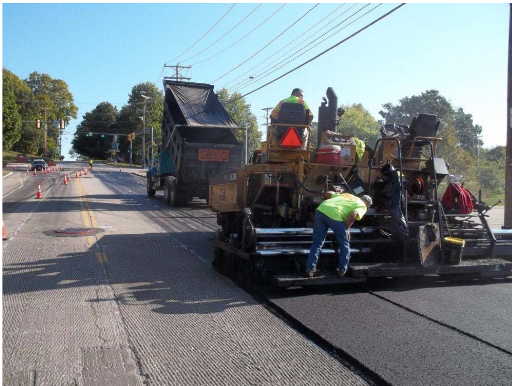
A Roadway Being Paved
