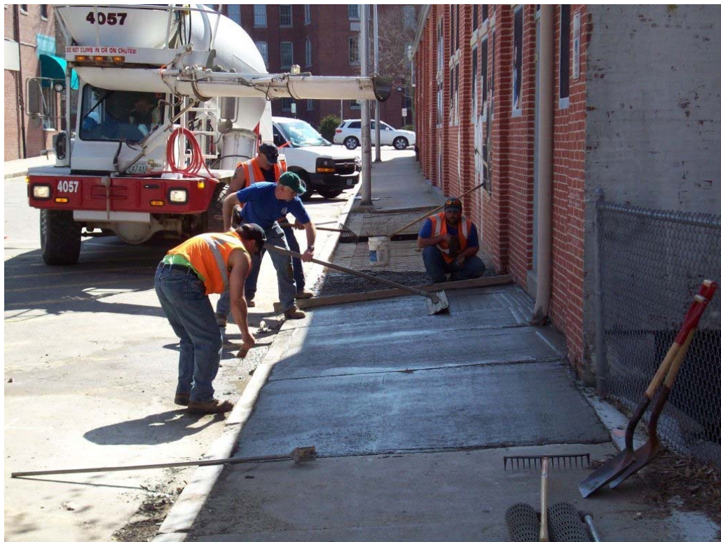
A Sidewalk Being Installed
