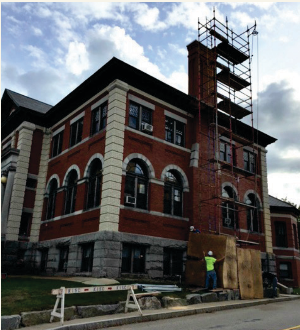
The picture on the left shows contractors in the middle of the Dover Public Library chimney repair project.
