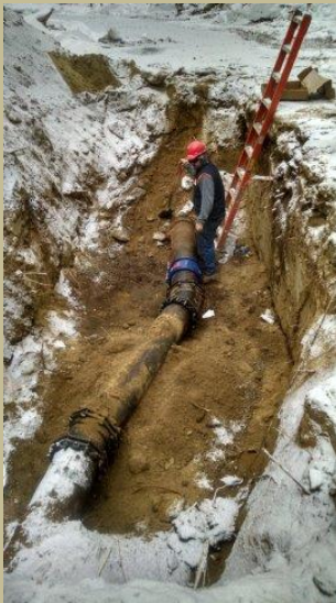
Zac Cole at Smith Well installing a new main.
