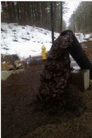
12" main pigging operation
