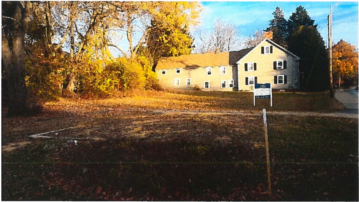
Photo 3: Looking northeast from corner of property at Central Ave and Merry Street.
