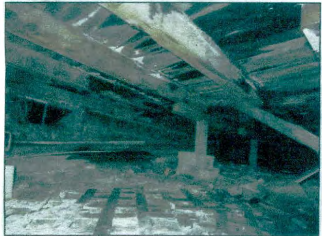
Leaning support posts on top of concrete blocks
