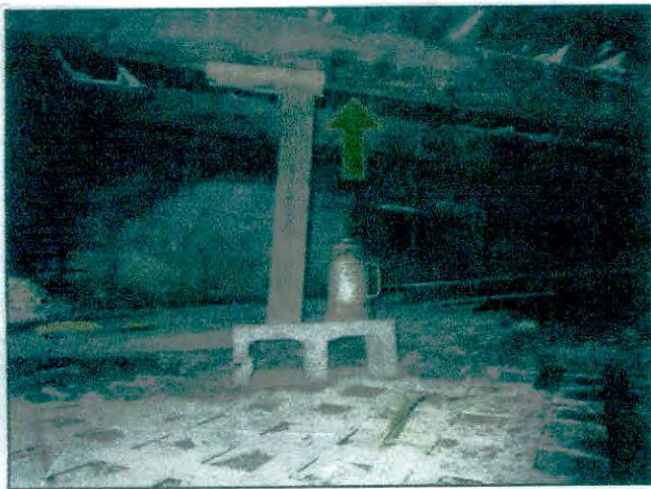
Leaning support posts on top of concrete blocks
