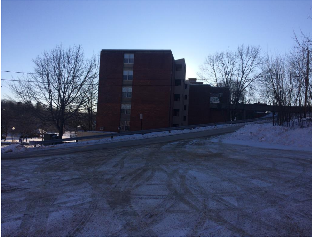
PHOTO #1: LOOKING SOUTHEASTERLY ACROSS WILLIAMS STREET AT APARTMENT BUILDING.
