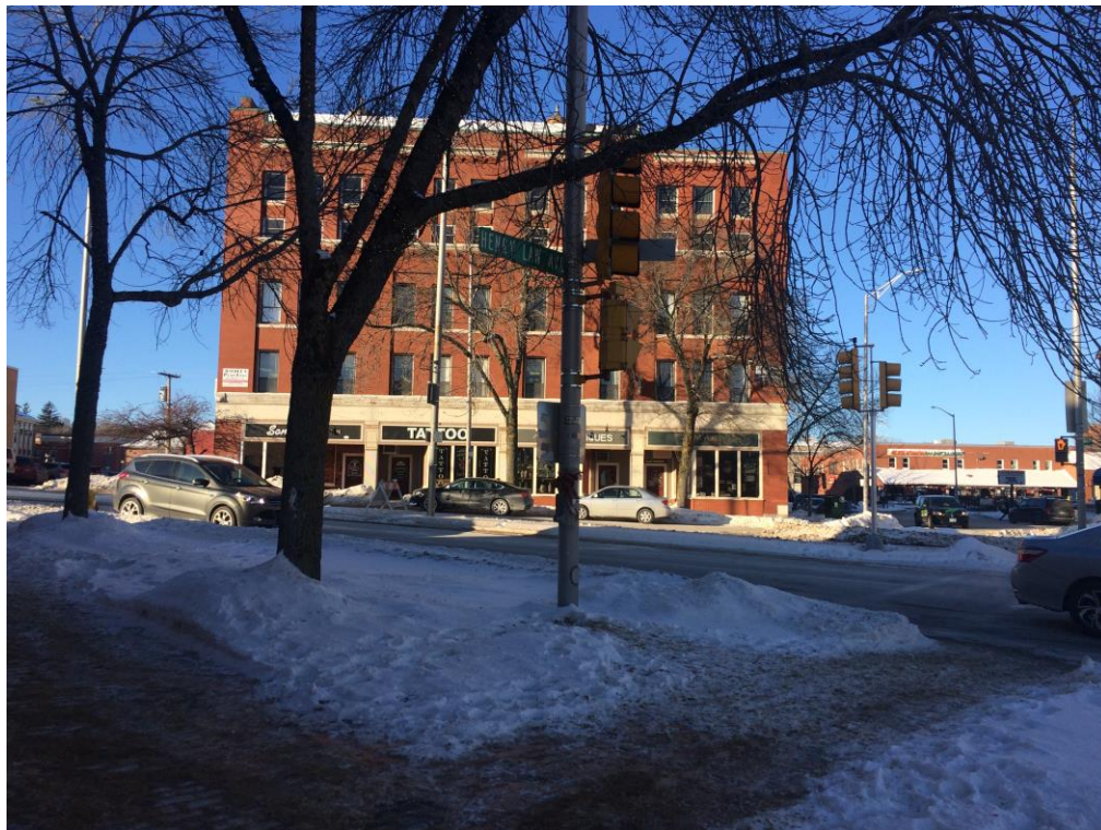
PHOTO #6: LOOKING WESTERLY ACROSS CENTRAL AVENUE AT A COMMERCIAL BUILDING.
