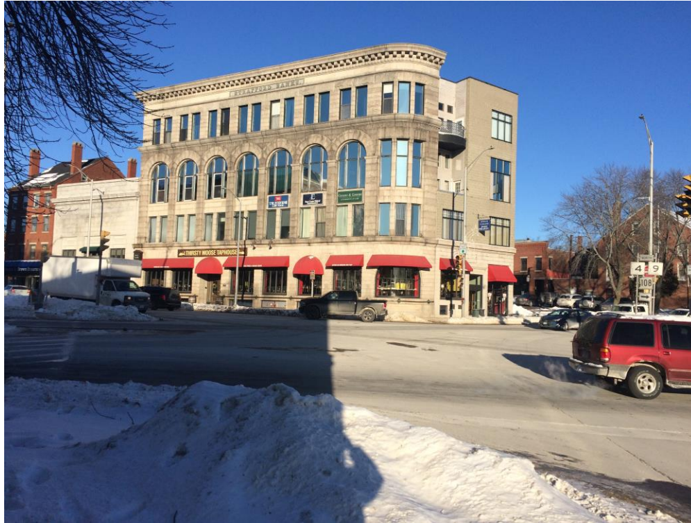
PHOTO #5: LOOKING NORTHERLY ACROSS INTERSECTION AT A COMMERCIAL BUILDING.
