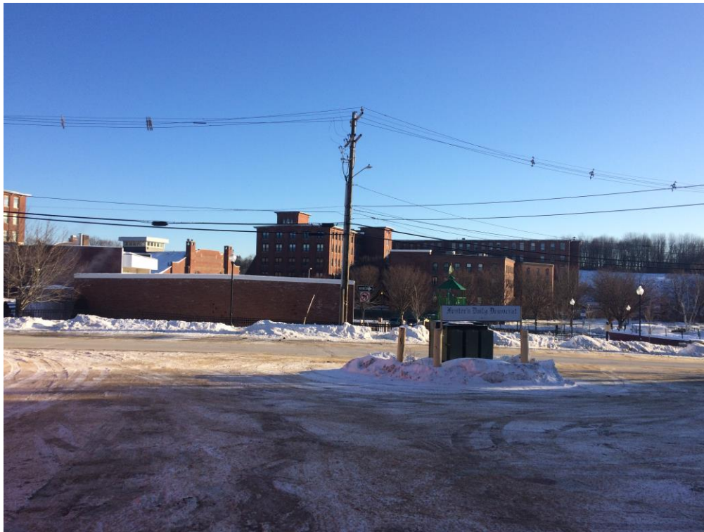
PHOTO #2: LOOKING NORTHEASTERLY ACROSS HENRY LAW AVE. AT HENRY LAW PARK AND THE MILLS BEHIND IT.
