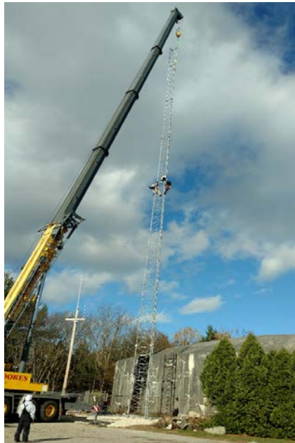
A crew from AllState Tower erects the 150' communications tower at the Garrison Hill Site
