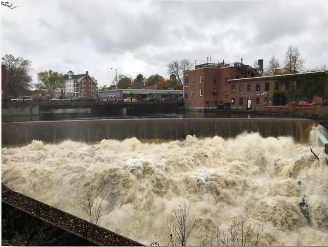
Cochecho River Dam, October 2017
