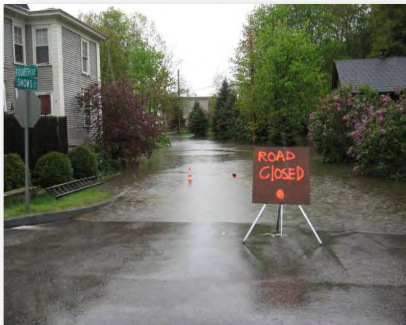
Flooding on the Snows Court, 2016
