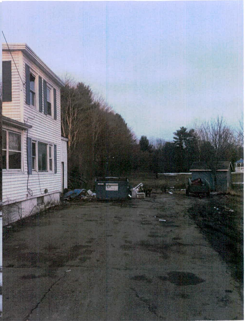
Existing Distressed Lot and Structure
