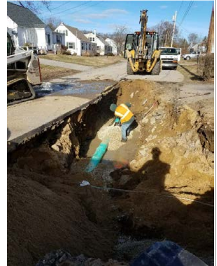
Eliot Circle Sewer Main
