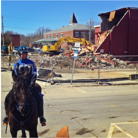
Above, Officer Caproni and Rasa check on the progress of the demolition of the Robbins building.
