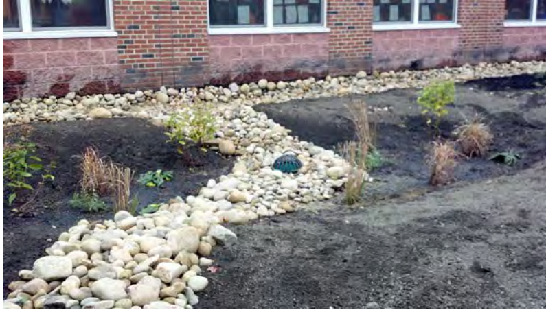
Figure 13: Horne Street Elementary School Bioretention 2 installed in October of 2011.
