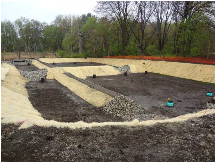
Figure 1: Subsurface Gravel Wetland located in headwaters of Berry Brook along south side of Central Avenue. Installation completed on May 2nd, 2012.
