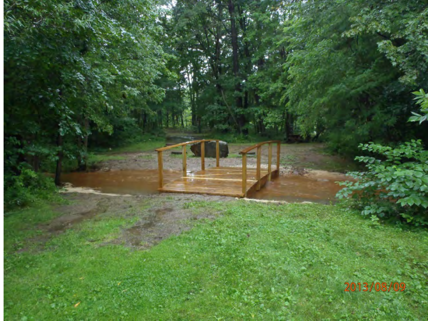
Figure 19: Station Drive Condominiums bridge installation that replaces a 12 inch culvert.
