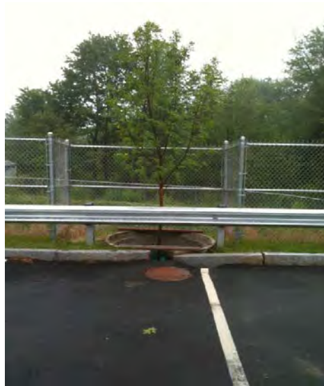
Figure 14: Horne Street Elementary School Tree Filter installed in June of 2011.
