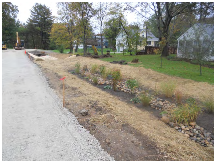
Figure 16: Snow Avenue Bioretention installed in September and October of 2011. Snow Avenue vegetated swale in the background.
