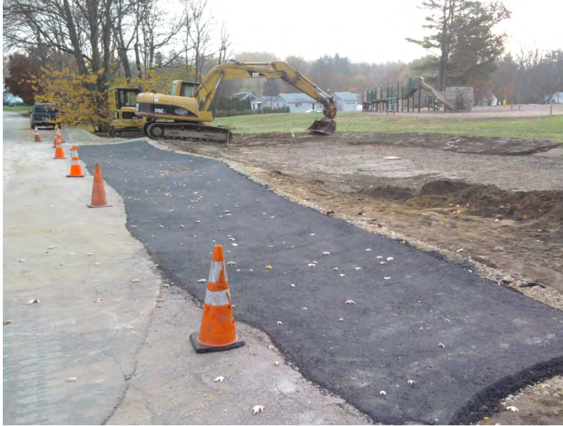
Figure 10: Glencrest Avenue Bioretention near completion installed in October 2012.
