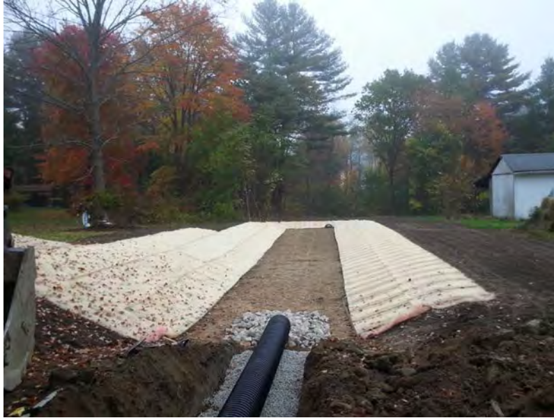
Figure 15: Horne Street Bioretention 2 installed in October of 2013.
