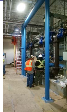
Above, sewer pump station staff attended a startup training for Lowell Avenue Water Treatment Facility.
