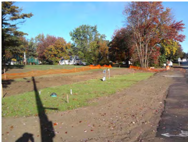
Figure 11: Upper Horne Street Bioretention installed in September of 2012.
