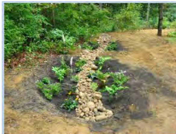
Figure 18: Hillcrest Drive Residential Rain Garden installed in October of 2011.
