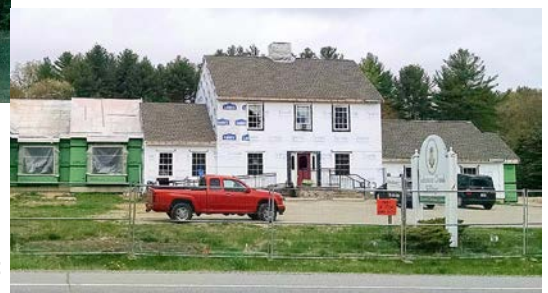
Pictured right is Johnson Creek Assisted Living project
