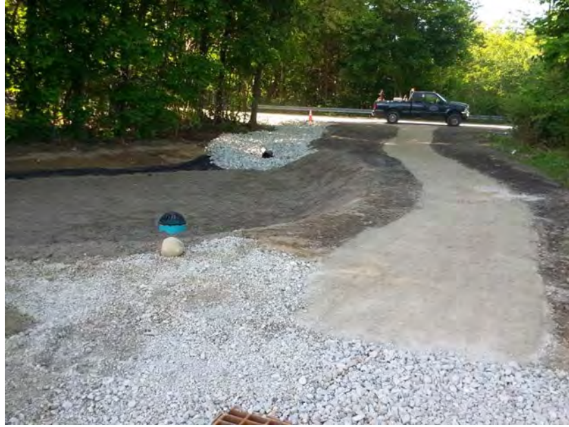
Figure 8: Roosevelt Avenue Bioretention and pedestrian pathway. Bioretention is too the left in the above picture. Construction completed in June 2014.
