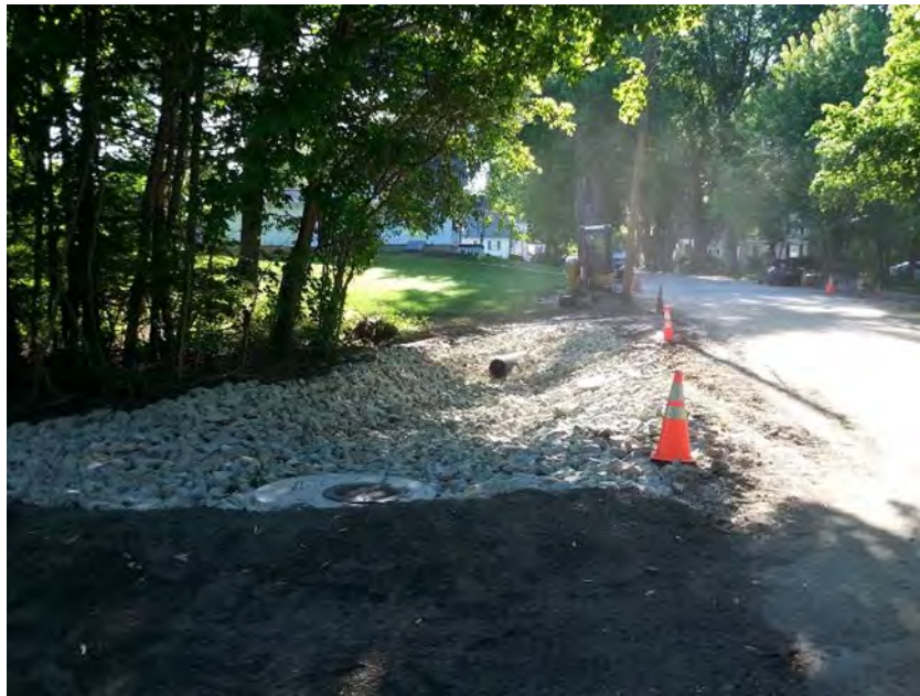
Figure 7: Roosevelt Avenue Rock Infiltration Basin installed off the north side of the road.
