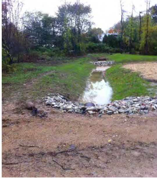
Figure 3: Page Avenue Vegetated BioSwale installed in September of 2011.
