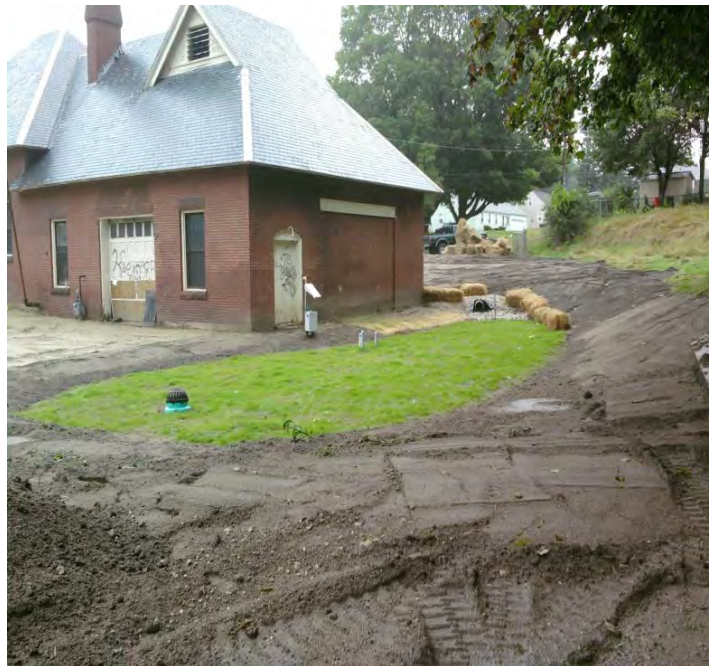
Figure 6: Lowell Avenue Bioretention installed in July through September of 2012.
