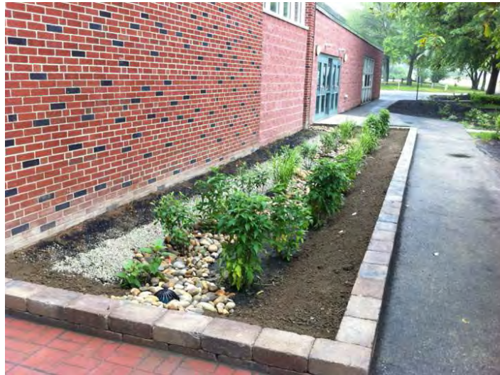
Figure 12: Horne Street Elementary School Bioretention 1 installed in June of 2011.
