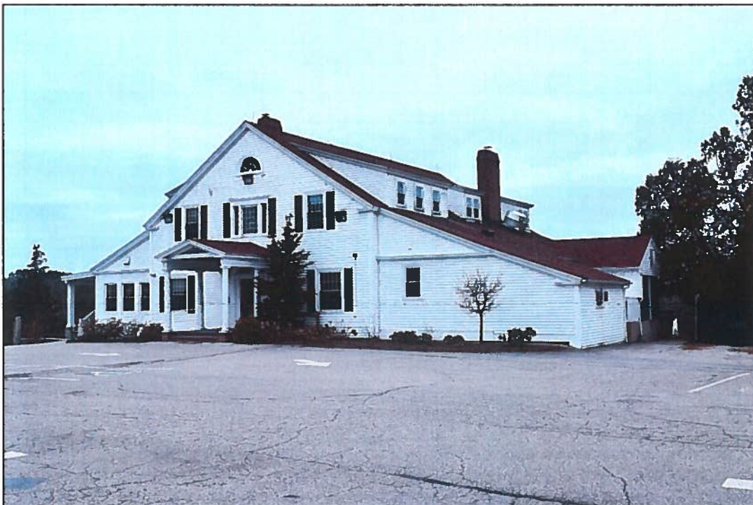
Photo 6. Cochecho County Club – Club House, 145 Gulf Road, view southwest.
