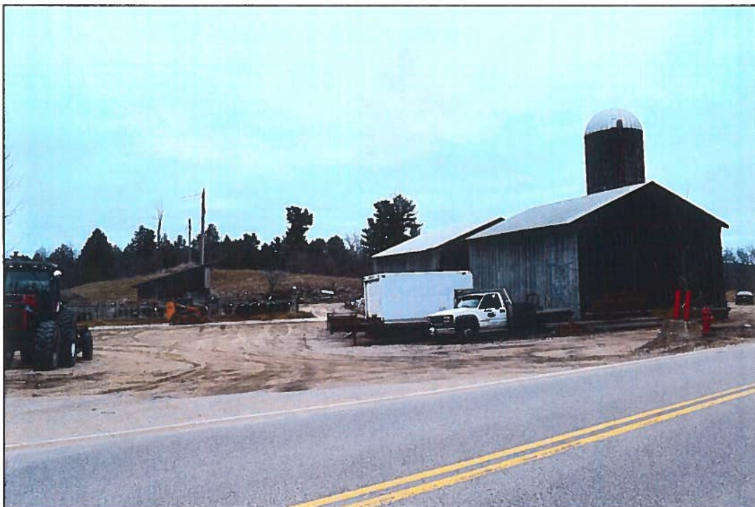
Photo 10. View northeast toward Project site and outbuildings on the Samuel Hanson II-Rousseau Farm property.
