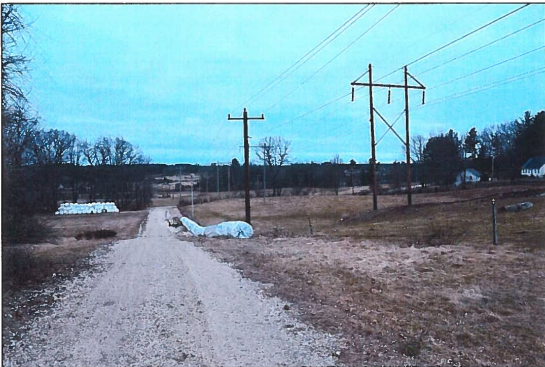
Photo 4. View south along access road from Samuel Hanson II – Rousseau Farm, showing location of transmission and gas lines and radio towers.
