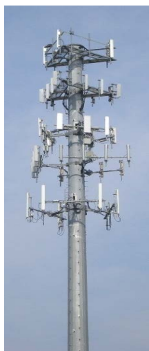
Non-Flush Mount Install
