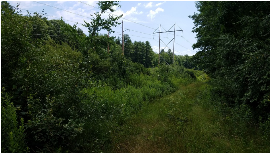
Figure 3. Access road toward Structure #51, at wetland DRW1 and ephemeral stream DRS1 crossing, facing east. Stream was dry with no flow.
