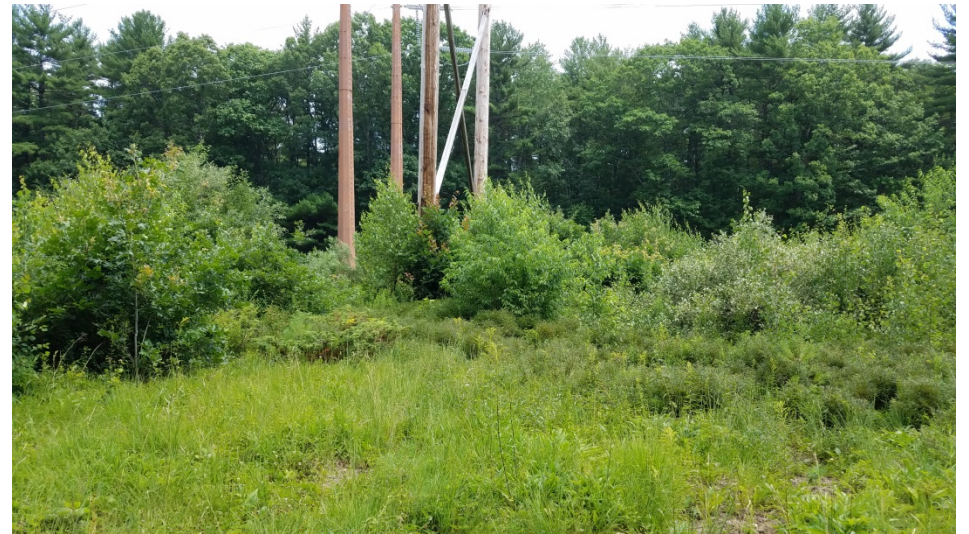
Figure 4. Structure #51; photo taken from access road, facing north.
