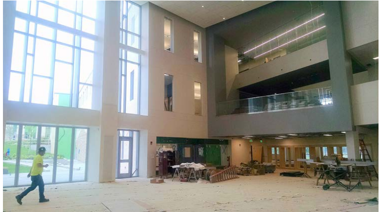
The above photo is of the new Dover High School; the town square area where students will eat lunch and congregate between classes.
