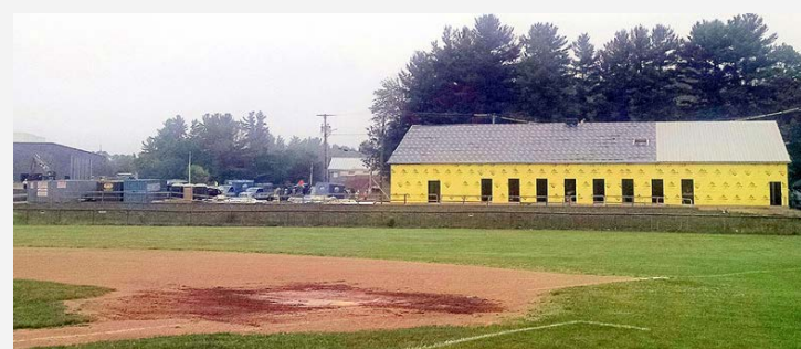
Pictured left is the work to date on the Animal Science Building on the campus of the new Dover High School.
