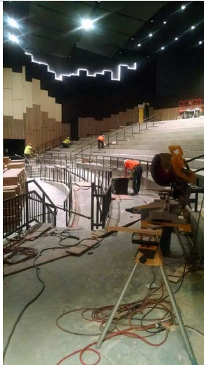
The photo to the left shows work in progress in the auditorium of the new Dover High School.
