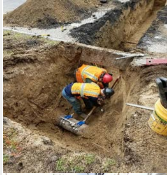
Shown left is a water crew tapping a water main.
