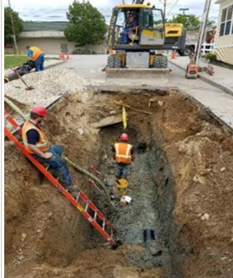
Shown left is the Ash Street trench.
